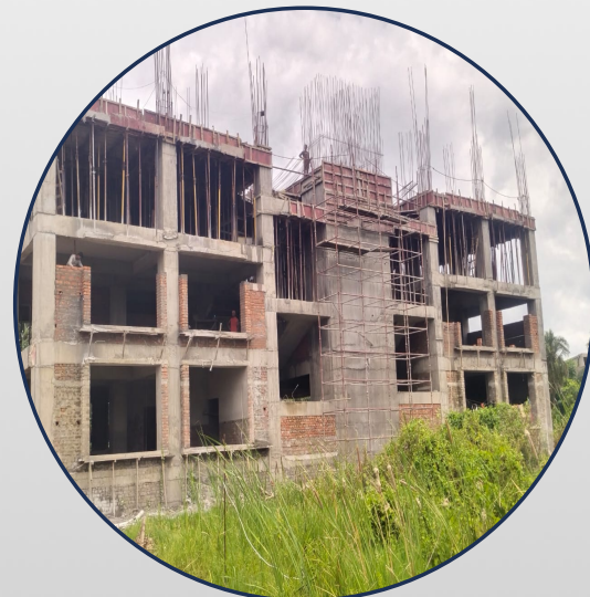
Netaji Subhas University of Sports & Entrepreneurship . University Block -II RCC frame structure, with finishing & MEP works. Approximate area 30000 square feet.
