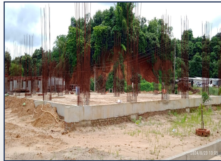
Techno India University, Tripura. Electrical Sub station 33 KV. Approximate area 2830.29 square feet.
