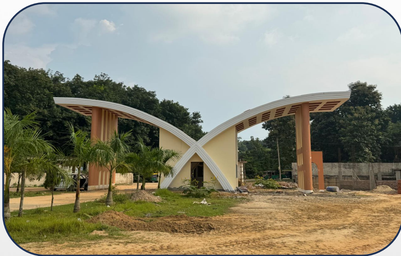
Techno India University, Tripura. Unique gate constructed with RCC structure.
