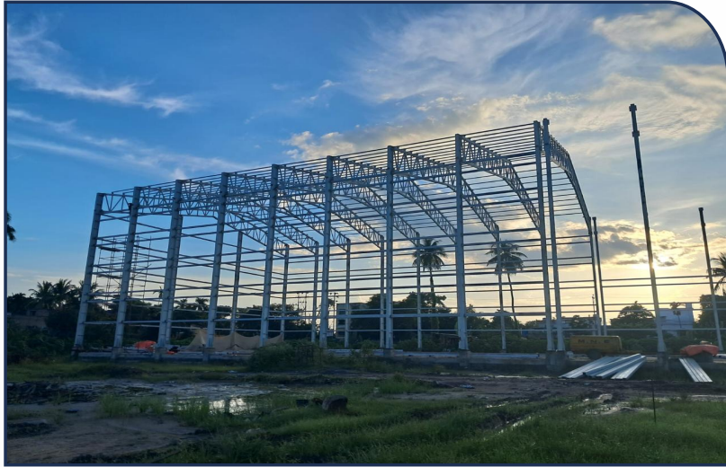
Netaji Subhas University of Sports & Entrepreneurship . Indoor stadium RCC foundation, MS frame structure building, with finishing & MEP works. Approximate area 25000 square feet. Structural steel 380MT, DGU 30000 square feet. ACP 32000 square feet. PUF Panelling 35000 square feet.
