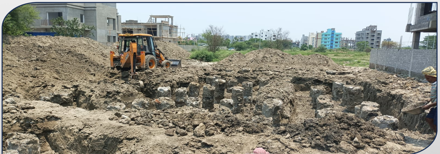
G+4 STORIED BUILDING 450MM Dia 18.00 meter dept Augure pile.
