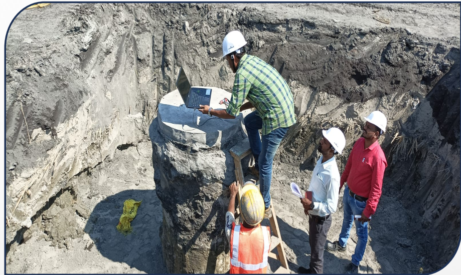
Piling work Switz Foods Pvt. Ltd. Location :- FP ¾, Food park III, Sankrail, Howrah Auger pile 300MM Dia 320 (approx.).
