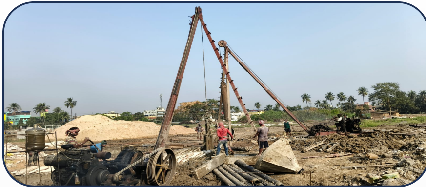
Sports University Chinsurah: 450MM and 600MM dia DMC Pile.
