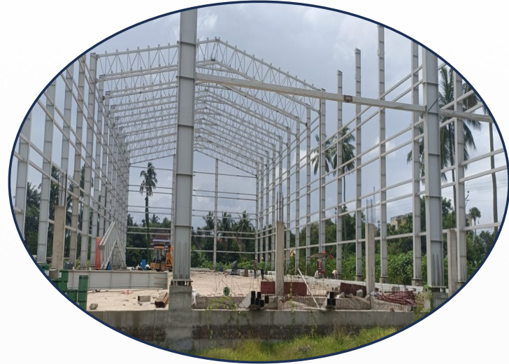
Netaji Subhas University of Sports & Entrepreneurship . Indoor stadium RCC foundation, MS frame structure building, with finishing & MEP works. Approximate area 25000 square feet. Structural steel 380MT, DGU 30000 square feet. ACP 32000 square feet. PUF Panelling 35000 square feet.
