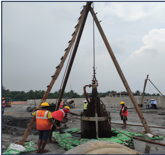
Piling work Switz Foods Pvt. Ltd. Location :- FP ¾, Food park III, Sankrail, Howrah Auger pile 300MM Dia 320 (approx.).
