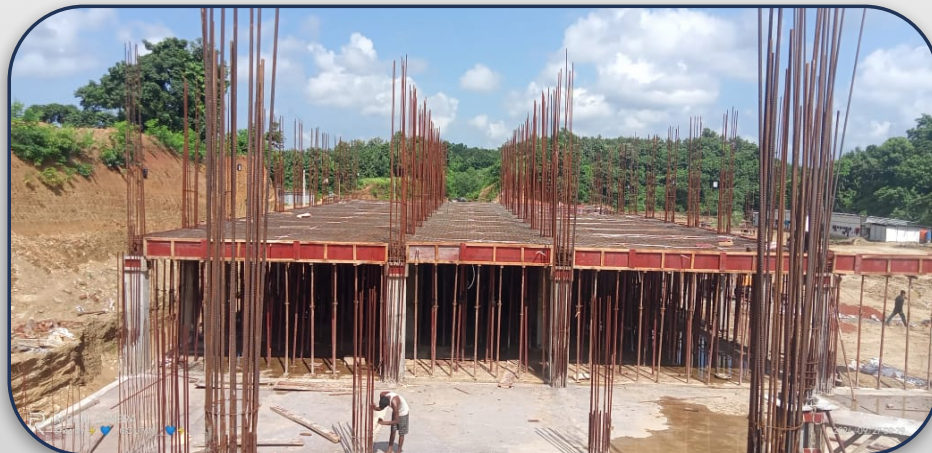
Techno India University, Tripura. Block-E - G+2 RCC frame structure building, finishing, HVAC, electrification low and high side, PHE. data Networking, CCTV, fire fighting works. Approximate area 65,000.00 square feet. Work in progress.
