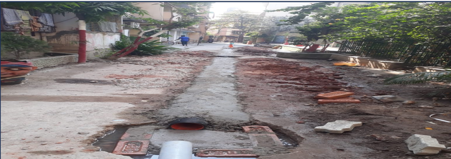
Binayak plumbing & drainage work
