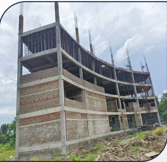
Netaji Subhas University of Sports & Entrepreneurship . University Block -I RCC frame structure, with finishing & MEP works. Approximate Area 48000 square feet.
