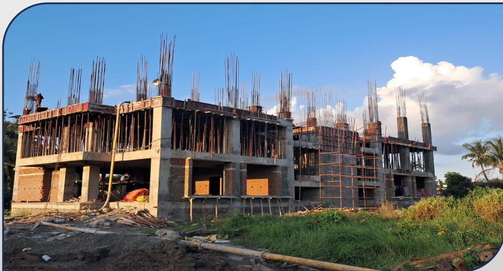
Netaji Subhas University of Sports & Entrepreneurship . University Block -II RCC frame structure, with finishing & MEP works. Approximate area 30000 square feet.
